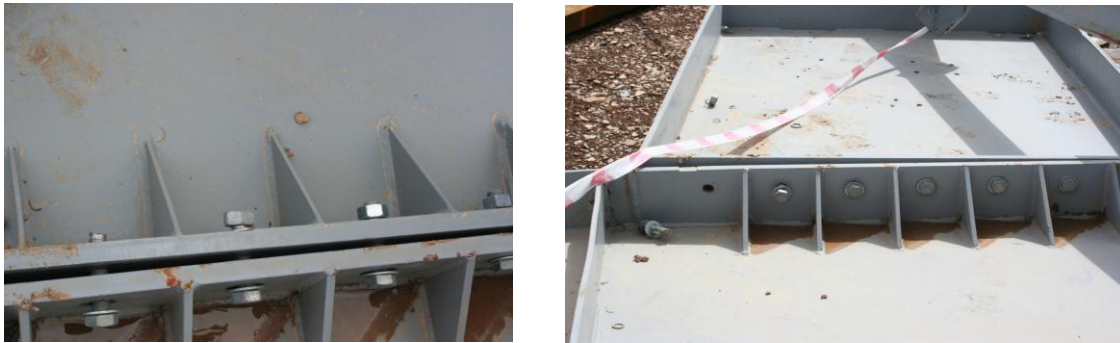
FIGURE 12. Snug Tight Connection During Construction
