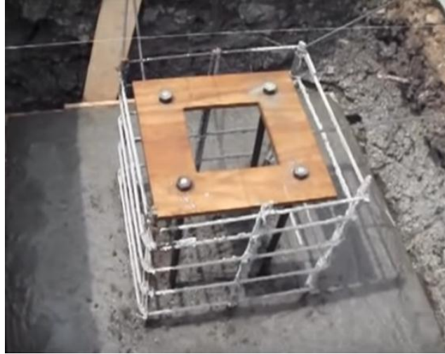
FIGURE 17. Typical Common Practice Pedestal Construction
