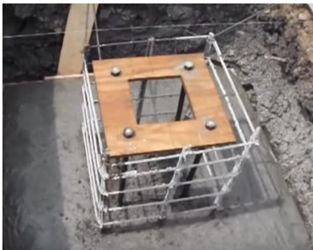
FIGURE 17. Typical Common Practice Pedestal Construction
