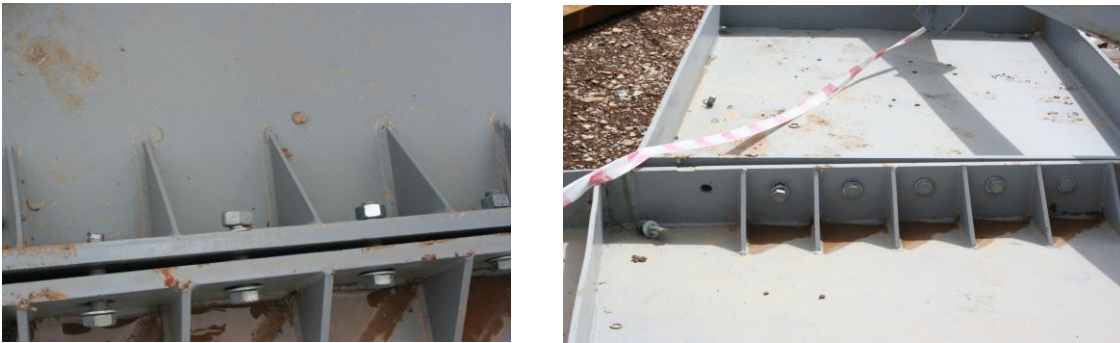
FIGURE 12. Snug Tight Connection During Construction
