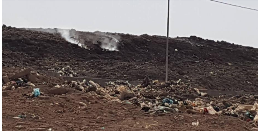
FIGURE 5. Gas emission from ELS (5 November 2017)
